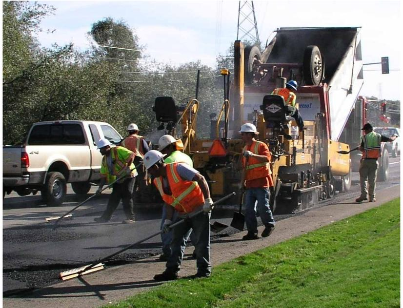
*Damaged roadway on Folsom Auburn Road is being removed and replaced in preparation for a Rubberized Asphalt Concrete overlay that reduces traffic noise.*
